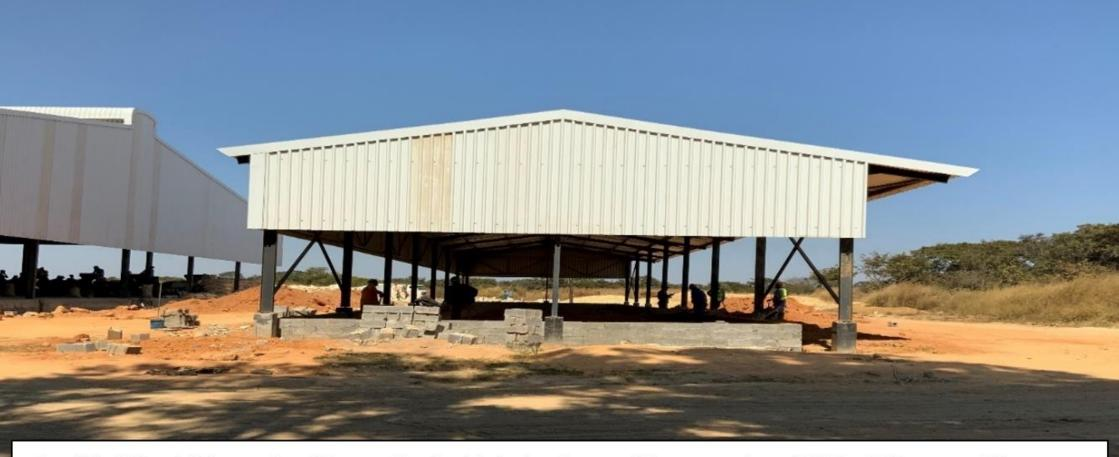
Zambia Mkushi Farms Seed Dryer Shed - 14 drying bays with a capacity of 150 – 200mt weekly. Remaining works include raising walls of the drying bays and installation of the heat source.
